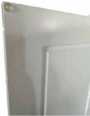
Full overlay framed doors with painted UV cured finish with reverse recess center panel
