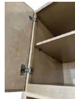
3/4" plywood full depth shelves with natural birch wood veneer finished and supported by metal pins.
