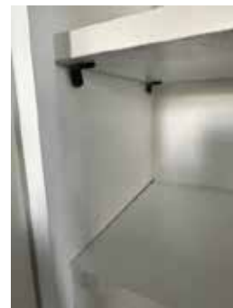
3/4" plywood full depth finished shelves with PVC edge banded on front and supported by metal pins
